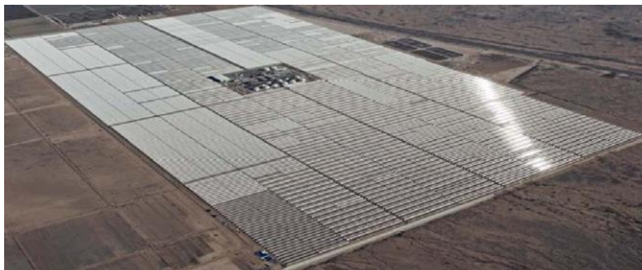
Fig. 10. Solana Generating Station. Power block and TES in the center (ABENGOA SOLAR, 2013).
