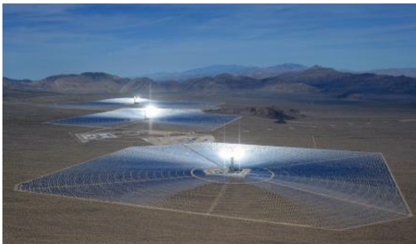
Fig. 6. Ivanpah Solar Power Tower facility (BrightSource Energy, n.d.)
