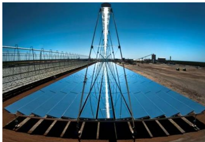
Fig. 9. Linear Fresnel Reflector from the Solar Down facility (Rajasthan, India) (AREVA Inc., 2012).
